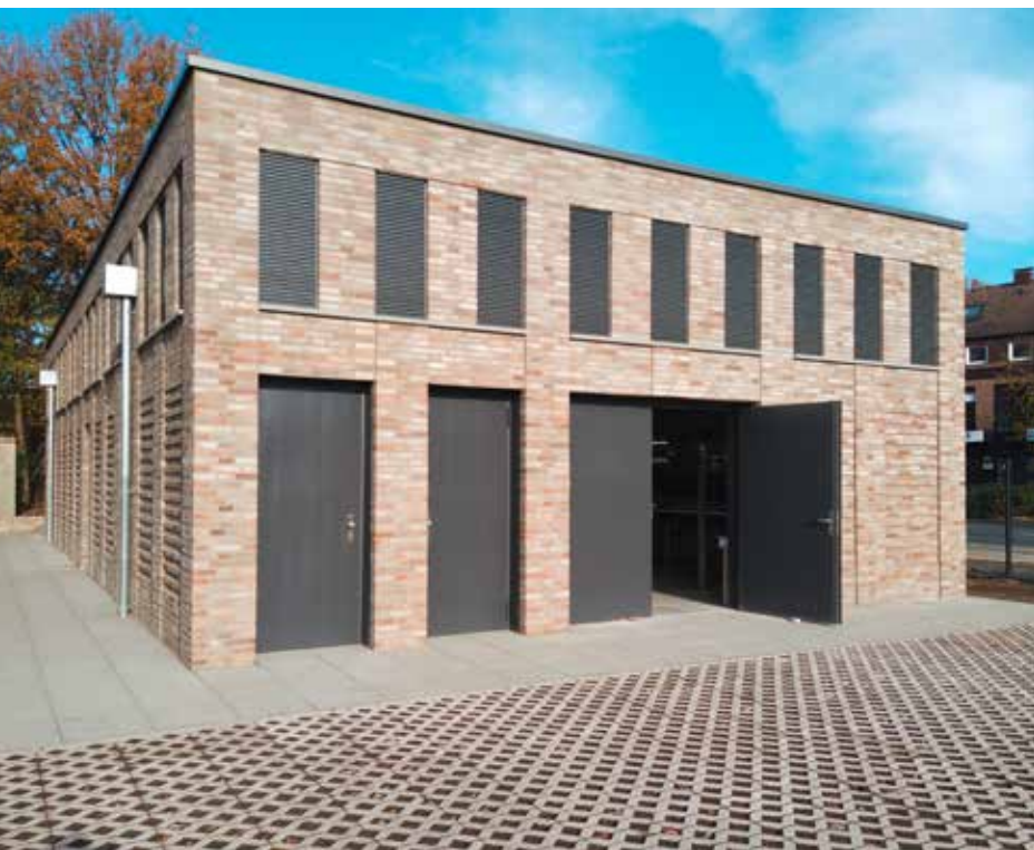
The boiler house for the York Quarter
