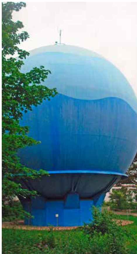
The gas sphere of Stadtwerke Gütersloh Photo: Hewa
